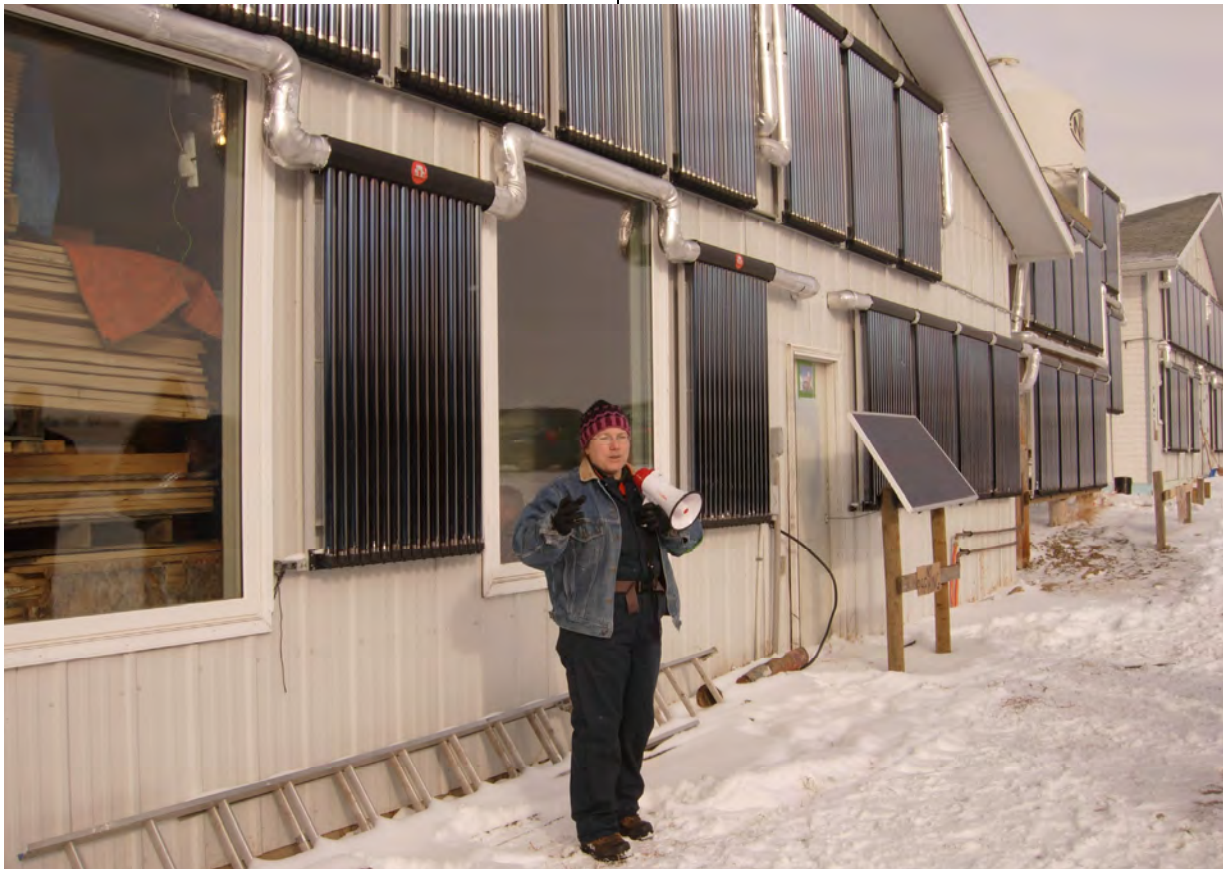
Photo: Karen Pedersen in front of the honey house. Evacuated tubes are mounted on the wall, and the photovoltaic panel is mounted on a stand next to the doorway. Karen would be happy to talk with anyone interested in their project – phone: (306) 398-3633 or email: karenpedersen@sasktel.net
